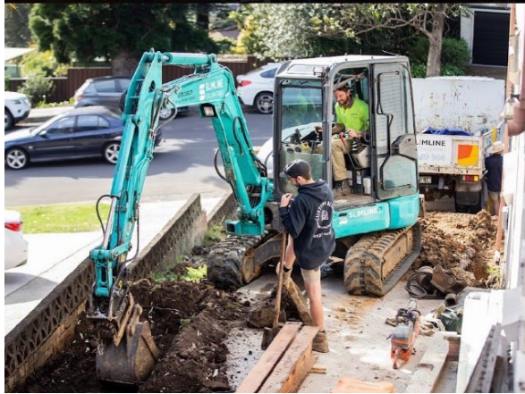
Slimline Excavations team busy at work
