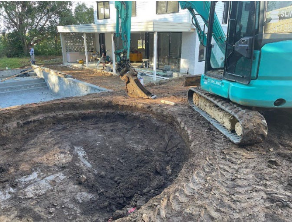
Finished, clean and tidy worksite using 5-tonne Kobelco excavator
