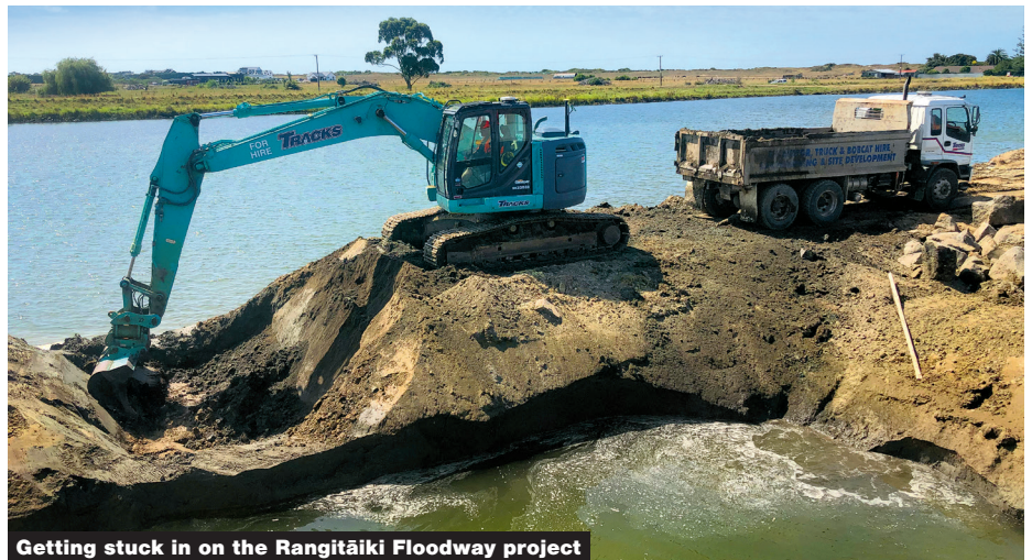
Getting stuck in on the Rangitāiki Floodway project
