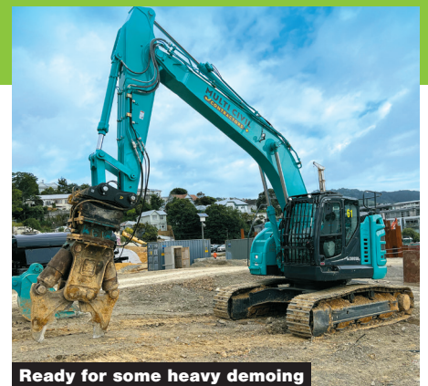
Ready for some heavy demoing
