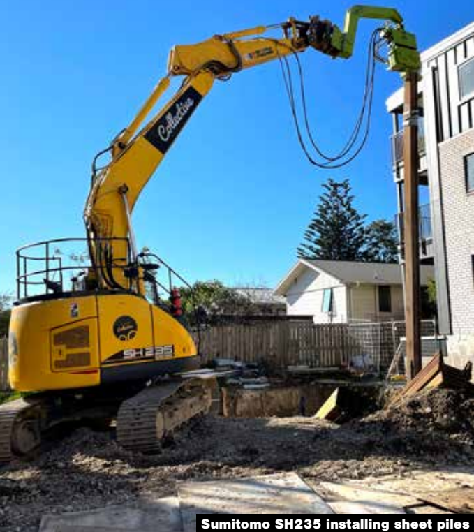
Sumitomo SH235 installing sheet piles
