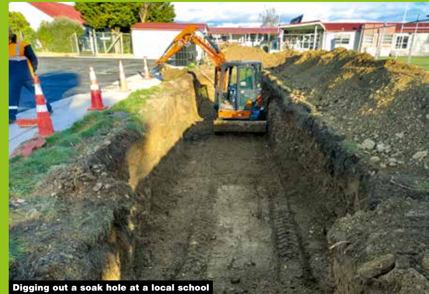
Digging out a soak hole at a local school
